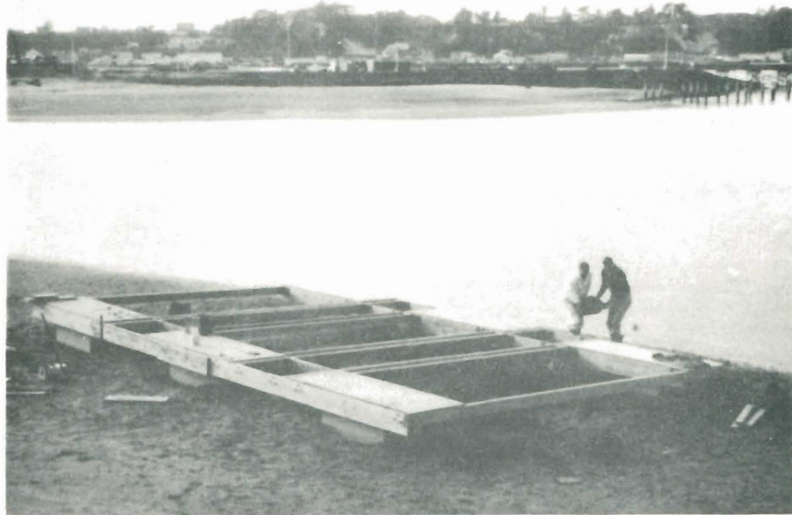
Figure 2. Oyster raft showing wood framework and fiberglass floatation units
