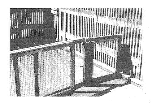
Clackamas Hatchery uses this crowder. It has an upper section that can be folded down as shown above allowing employee to easily crawl over or be raised as shown below while crowding fish, this preventing fish from jumping over.
