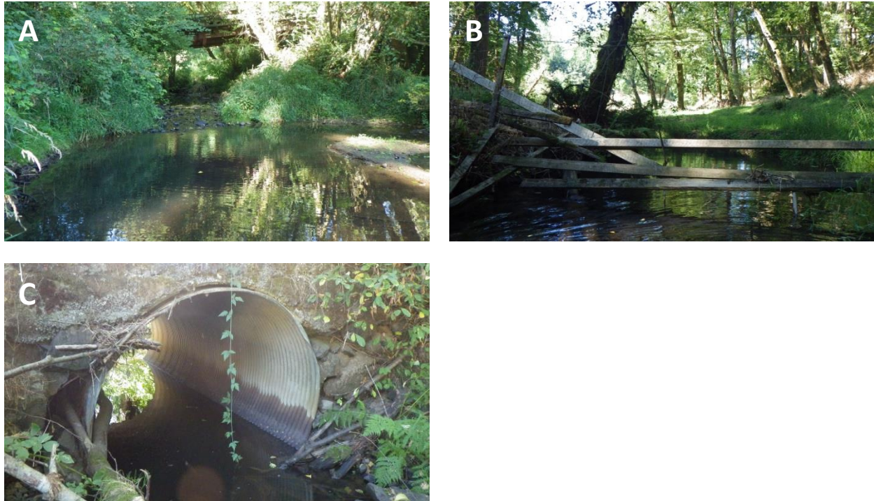
Figure 24. Survey pictures on reach 2 of Merrill Creek showing a private bridge (panel A), a broken cattle fence near the upstream end of the reach (panel B), and a circular culvert located under Hills Haven Road (panel C).
