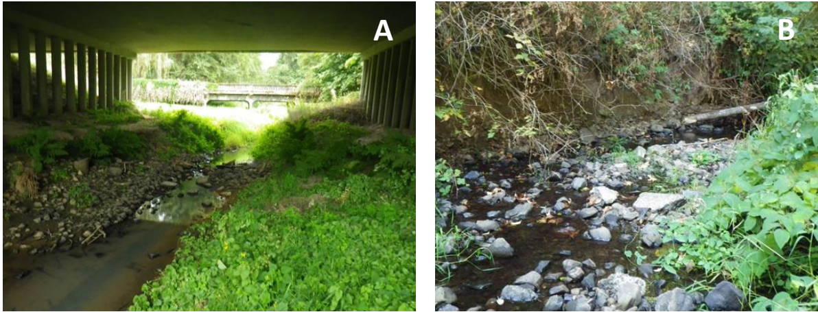
Figure 19. Survey pictures on reach 2 of McCarthy Creek showing the Highway 30 bridge at the downstream end of the reach (panel A) and invasive knotweed growing along the bank in the upper section of the reach (panel B).
