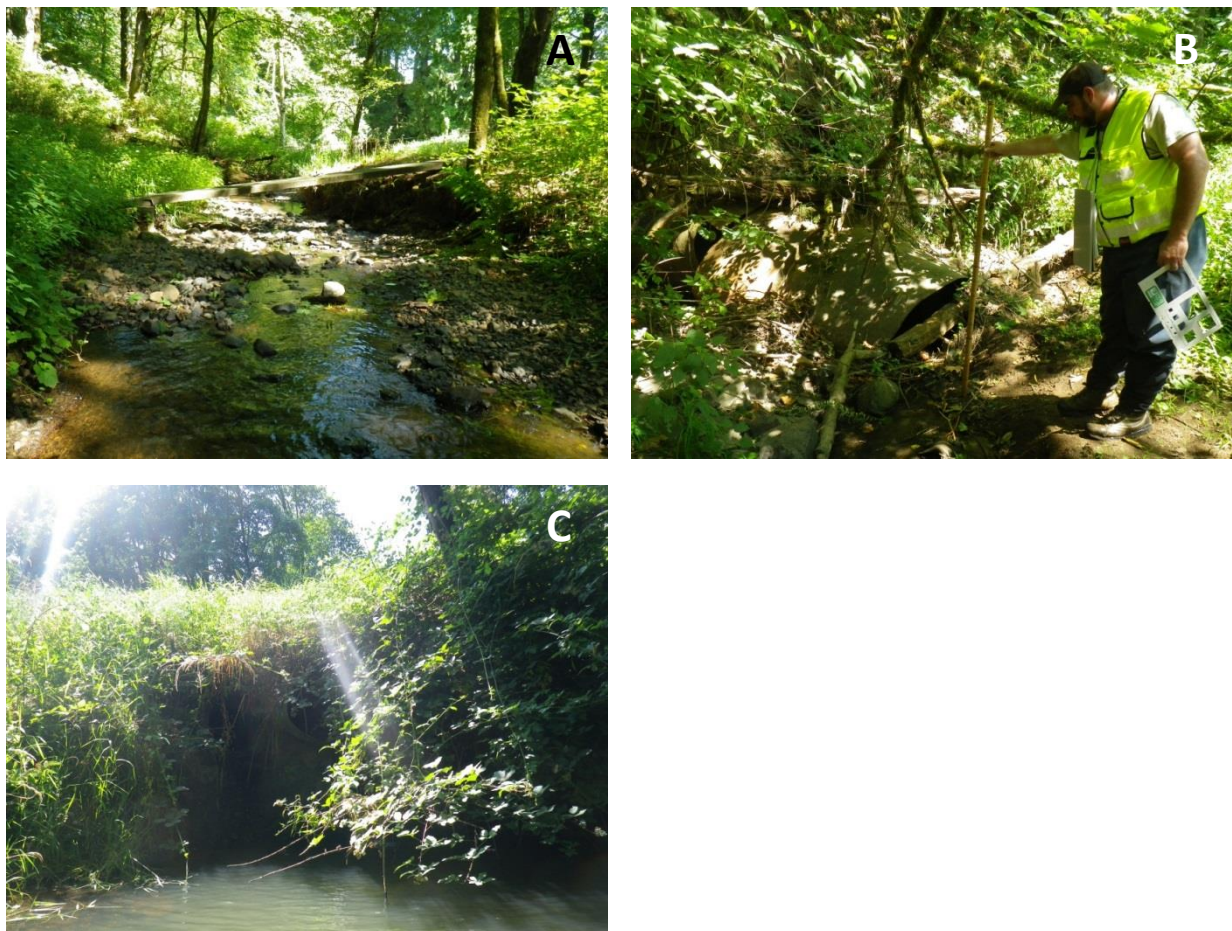
Figure 16. Survey pictures on reach 2 of McBride Creek showing a small footbridge (panel A), the lower culvert (panel B), and the downstream end of the double culvert at the top of the reach (panel C).
