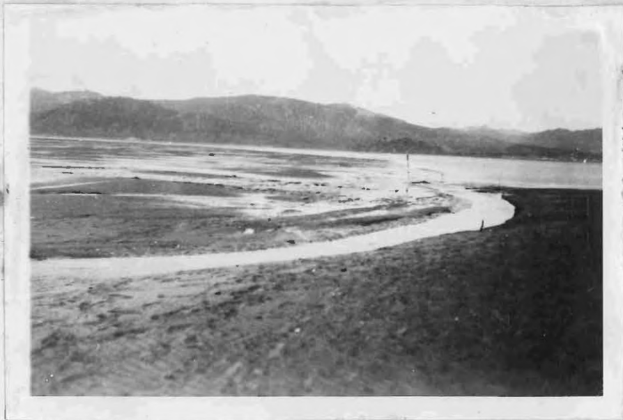
TEST AREA BEFORE BLAST
