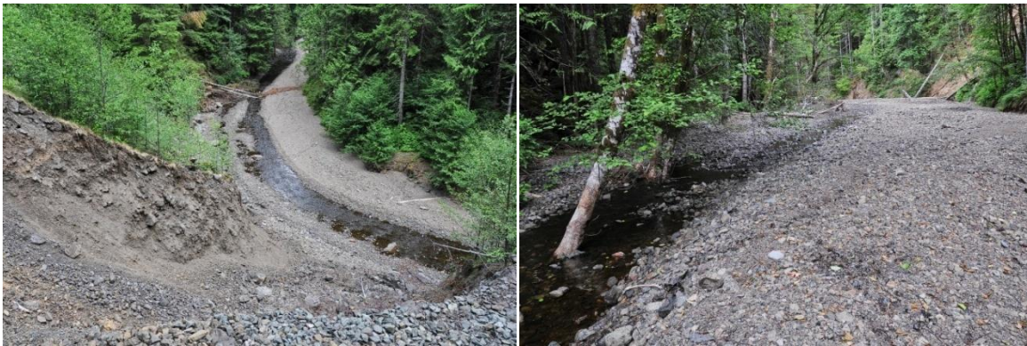
Fig 23 (left). Wolf Creek, July 2008. This slide, one of many short slides down the canyon sides, originated on the railroad grade. Fig 24 (right). Wolf Creek, July 2008. The creek subsides entirely into the gravel in the distance.
