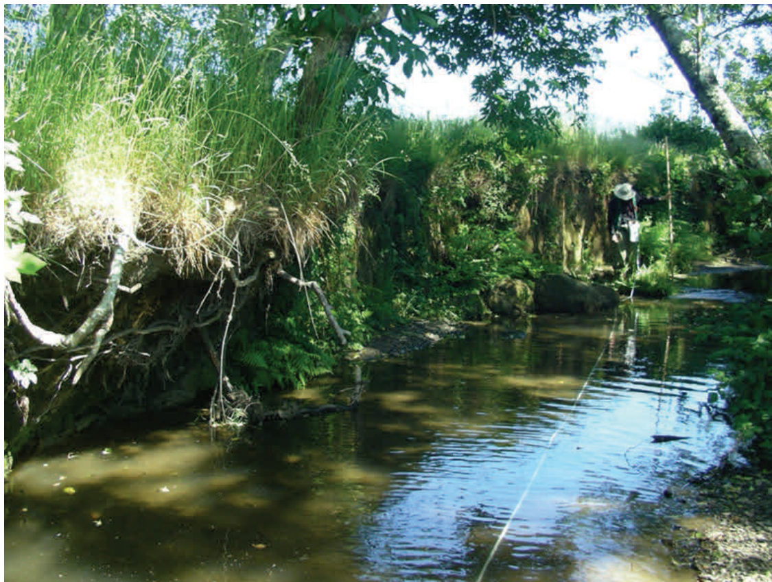
2008—Reach 2, unit 87: Looking upstream at a segment of incised channel that was modified in 2009 through the construction of inset floodplain terraces and bank sloping.
