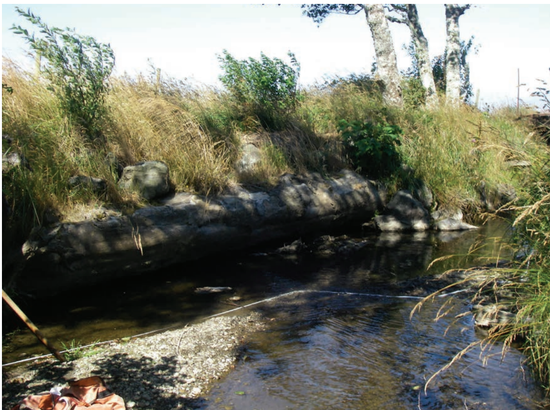
2012—Reach 2, unit 65: Looking downstream at the “cutoff” where the old channel was abandoned and filled — the log and rocks were used to seal off the old channel.
