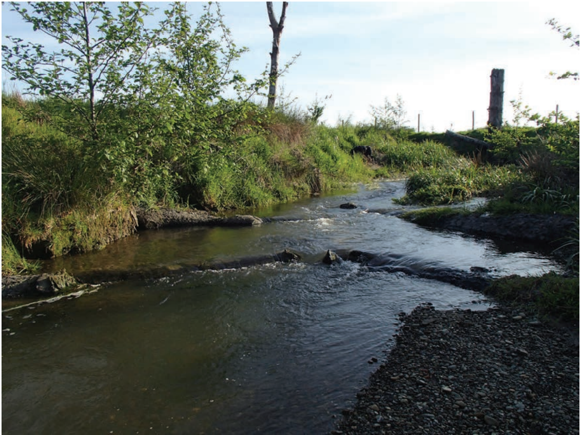
April 2014—Looking upstream at one of three log weirs constructed in 2011 for grade control to arrest and reverse the upstream migration of a headcut.
