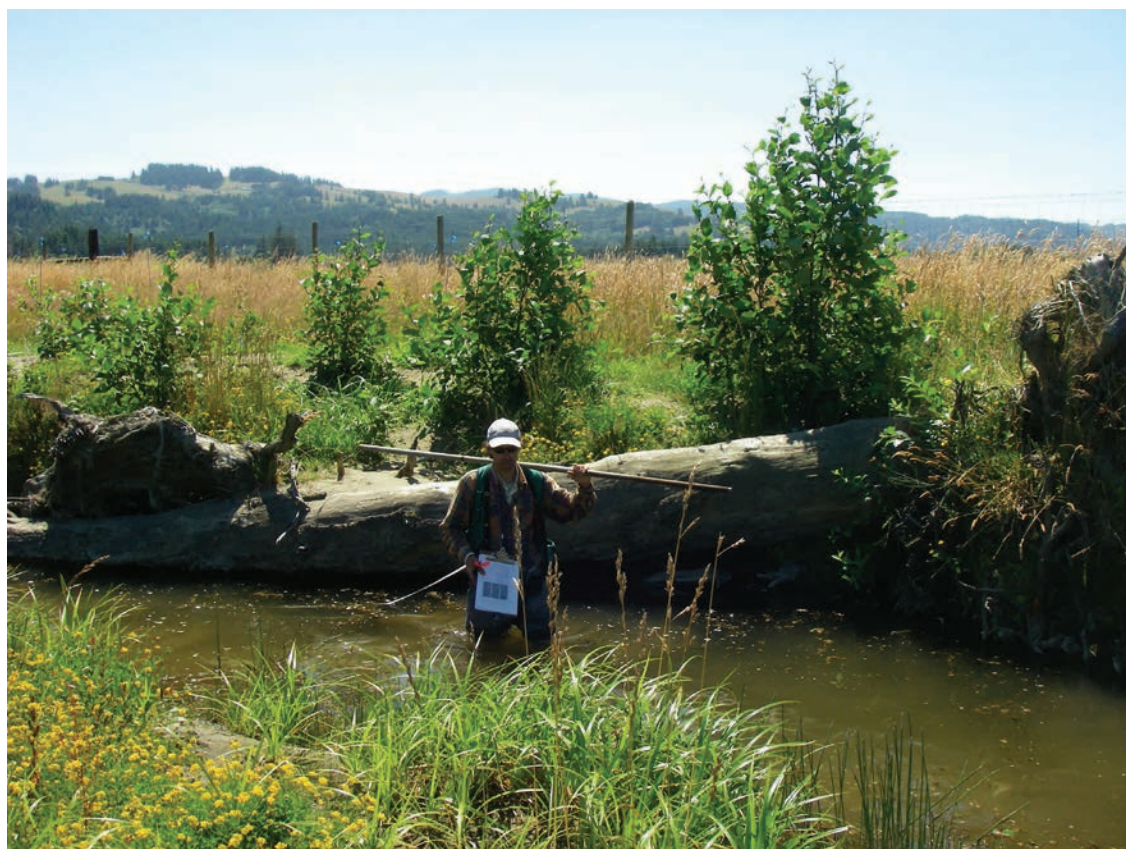
2012—Near the start of Reach 2, unit 15: Looking upstream on the new channel at a lateral scour pool and log structure.
