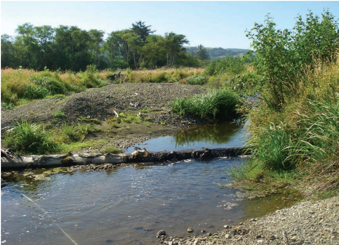
2012—Reach 2, unit 53: Looking upstream at the in-line sediment retention pond that was designed as a “sacrifice area” where incoming bedload could be removed to prevent the downstream channel from filling with sediment. In Year 1 ~200 cubic yards were removed, but no material has been removed since because USACE erroneously omitted bedload removal from the removal-fill permit authorization.
