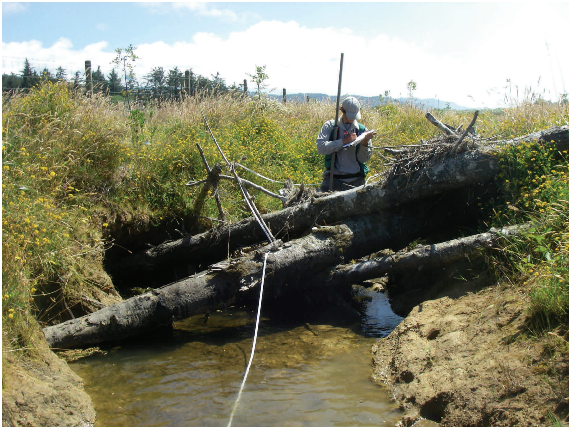
2012 Reach 2, unit 32, looking upstream at large wood placement within newly constructed channel reach.
