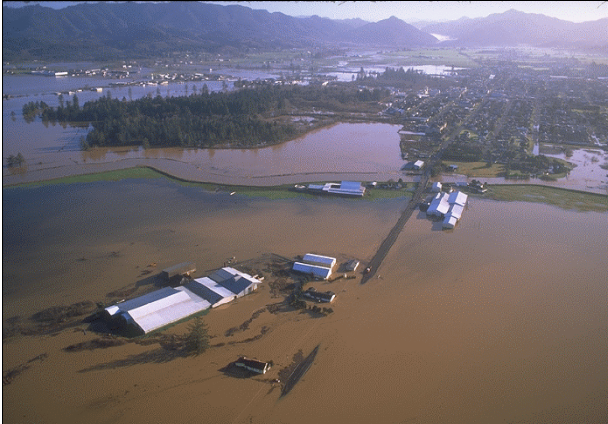
Figure 6-11. Aerial photograph of flooding on February 10, 1996, at Tillamook, OR. after the floodwaters had begun to recede.
