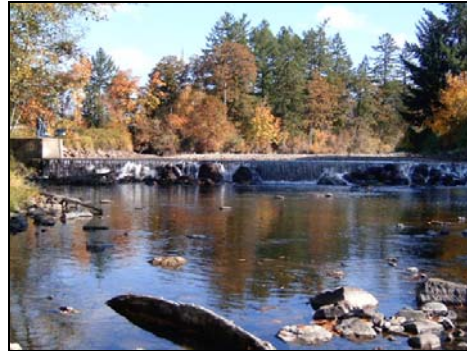
The Brownsville Dam was constructed as a hollow-core concrete dam.
