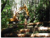
Figure 1 Constructed log jam on Big Creek
