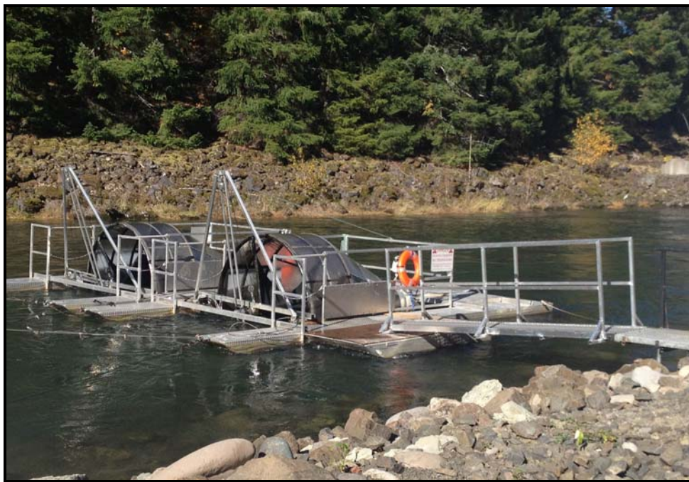
Figure 1. Turbine tailrace rotary screw traps (2.4 m diameter; rkm 385) below Cougar Dam.
