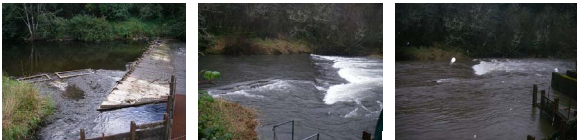
Figure 3. PIT antenna at Salmon River Hatchery weir. Left – low flow; center – moderate flow; right – high flow and still operating.
