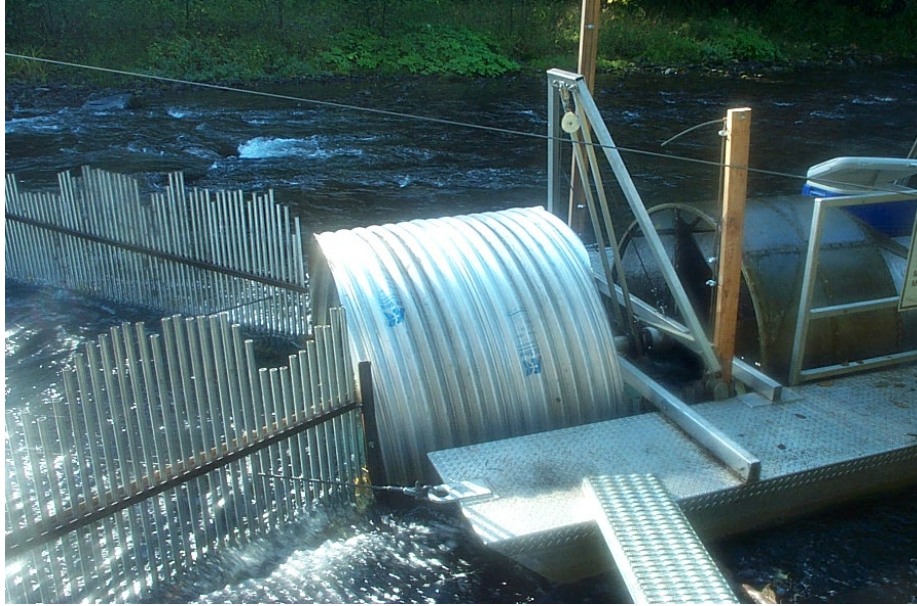
Photograph 2. We cut off the top half of the downstream portion of the culvert and the culvert extends downstream under the #1 and #2 beams of the screw trap to within about an inch of the trapping cone. The V-shaped weir extends from the upstream end of the 5-foot diameter culvert to within 5 feet of the bank.
