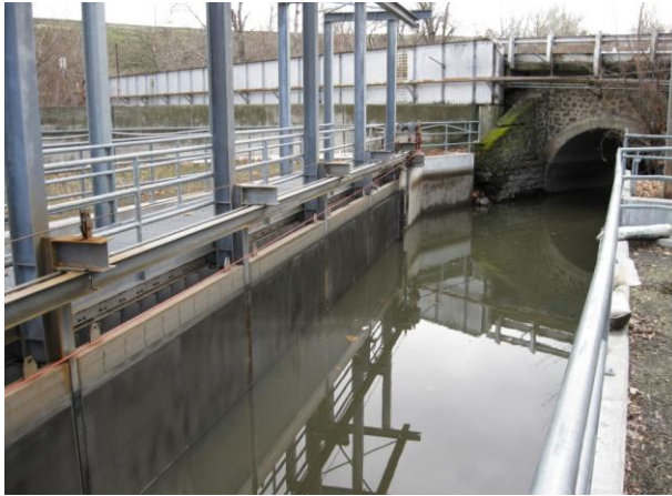
Fish screen forebay LWW headgate
