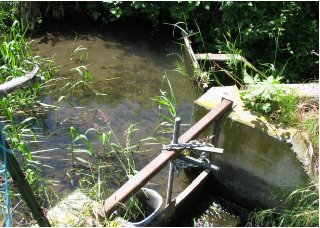
Typical Diversion in lower LWW
