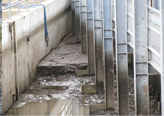
Clearing sediment from headgate fish screens
