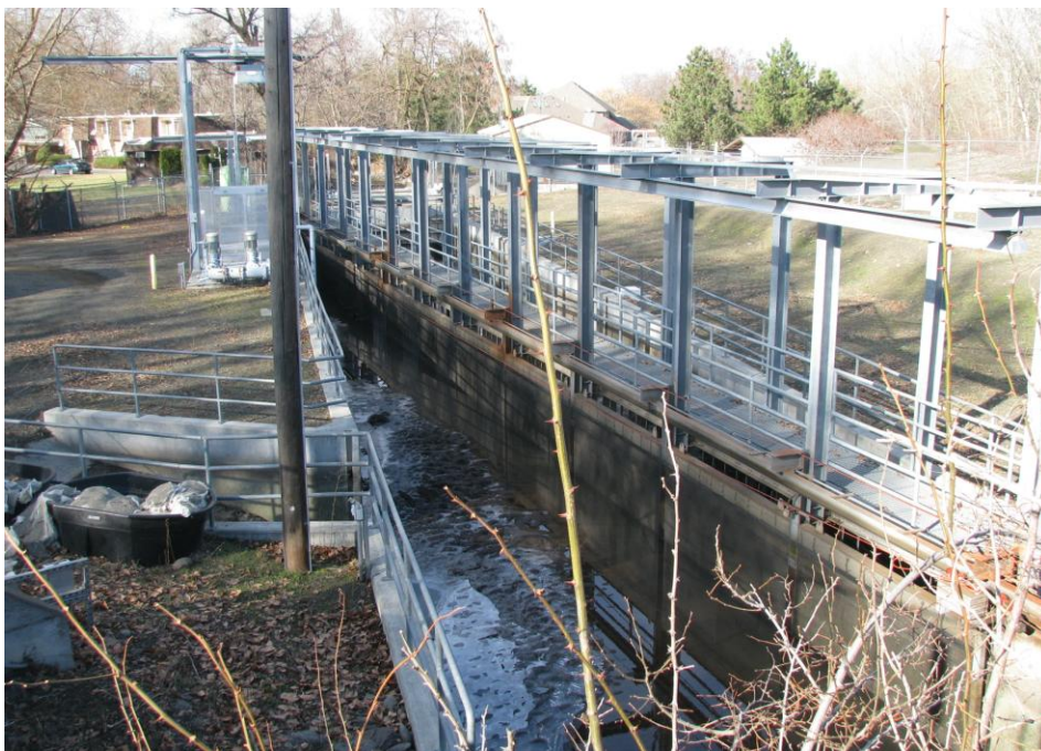
Little Walla Walla Fish screens shut down for winter maintenance
