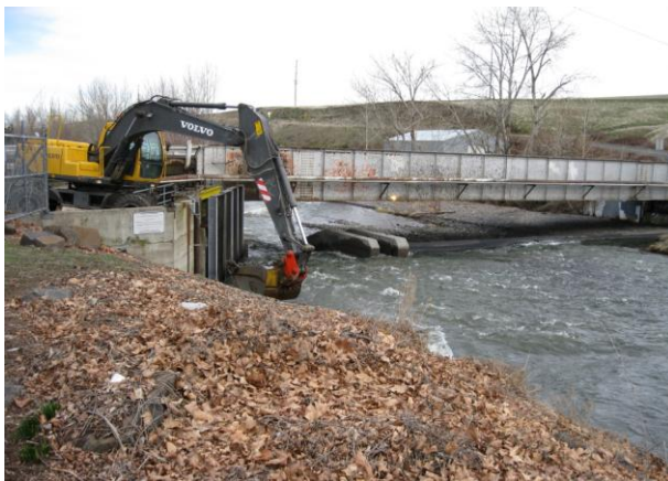
Clearing WW river gravel buildup at headgates
