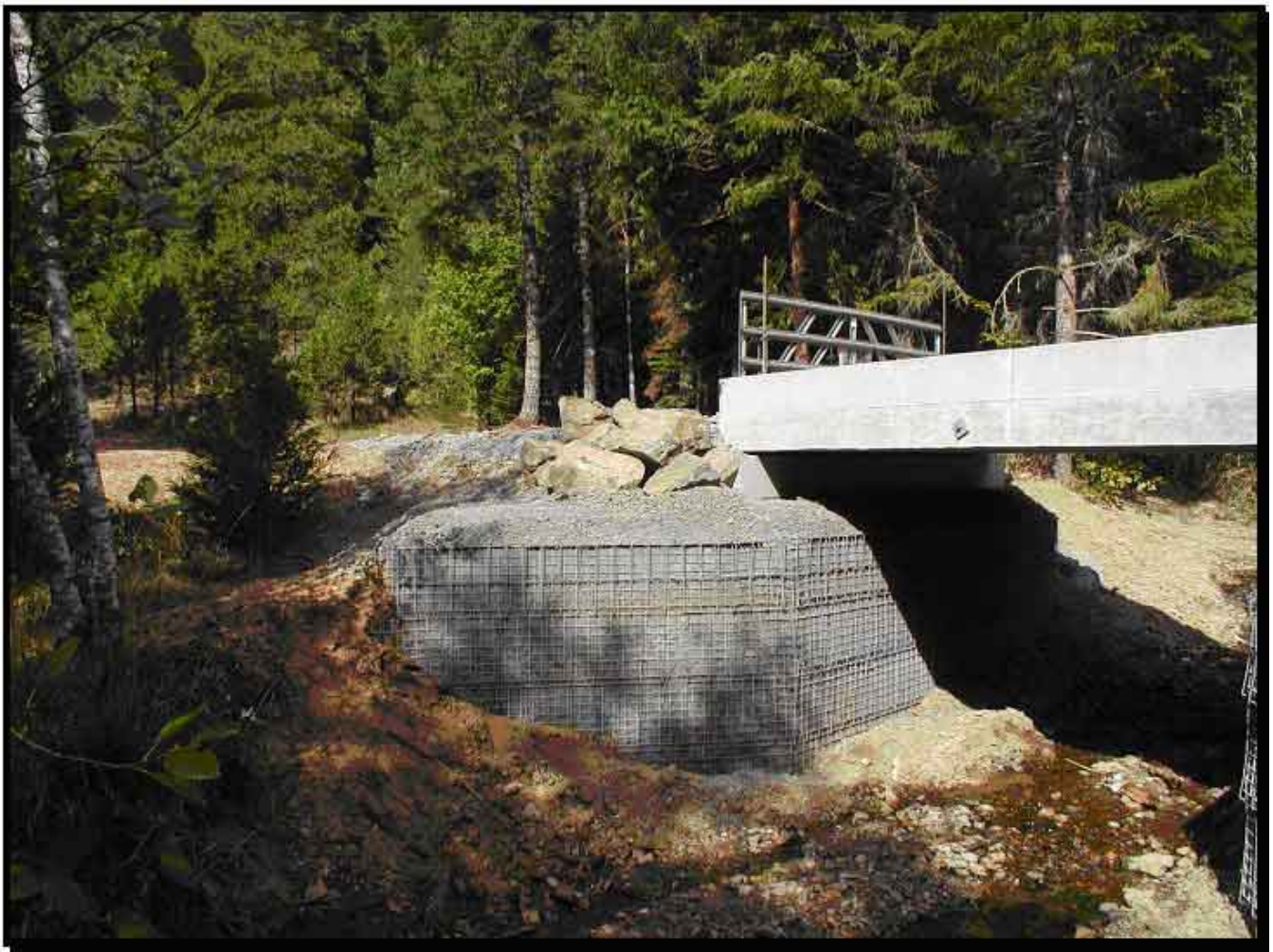
Figure 3 Hilfiker wall on west approach of bridge.
