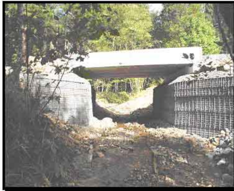
Figure 2 Completed project with Morse Bros. Bridge and Hilfiker walls
