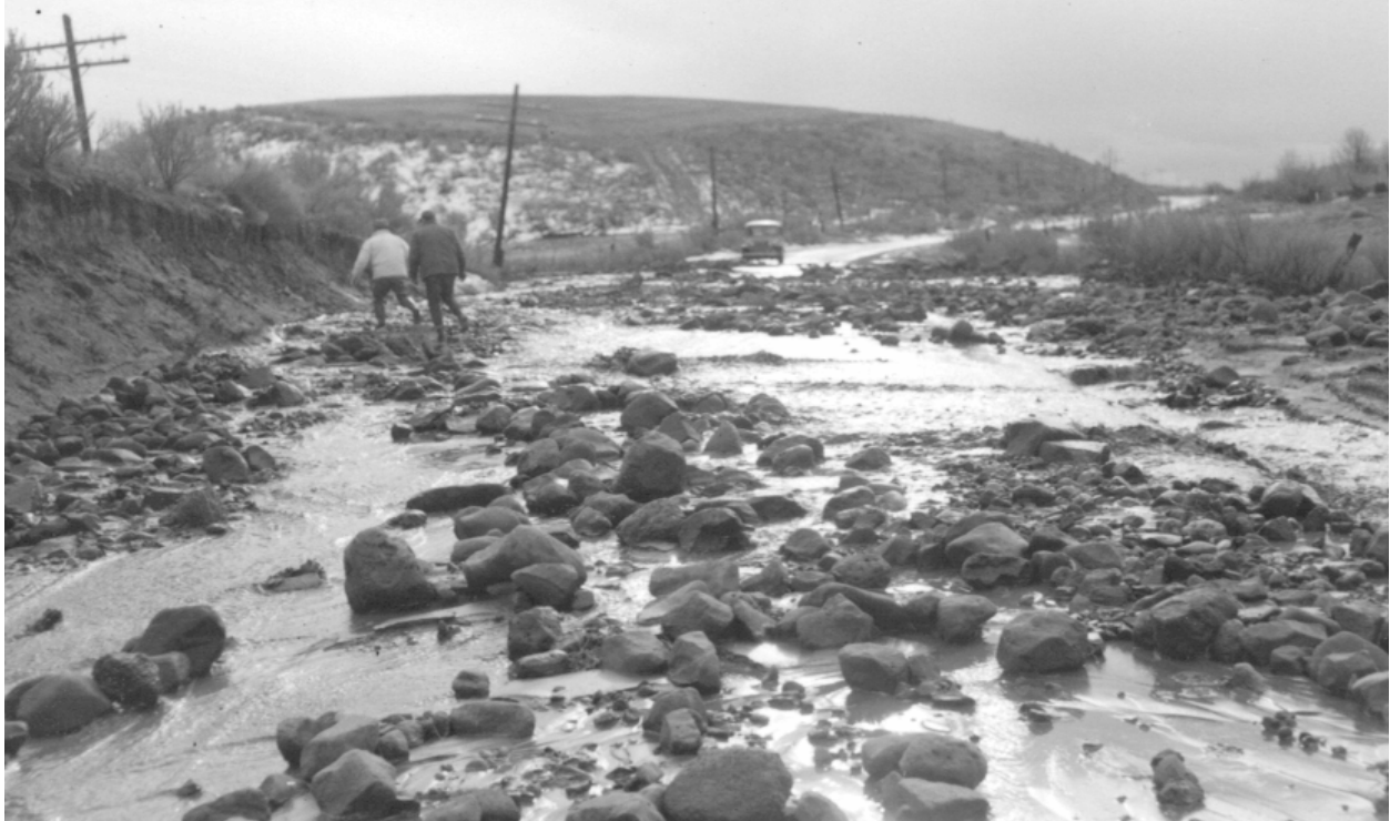
Figure 3.5. Boulders washed onto Highway 19 one mile south of Olex, Oregon, during the 1964 flood.
