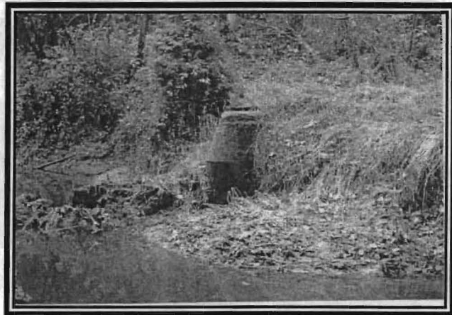
Figure 5. Municipal sewer line crossing Tryon Creek, reach 4.
