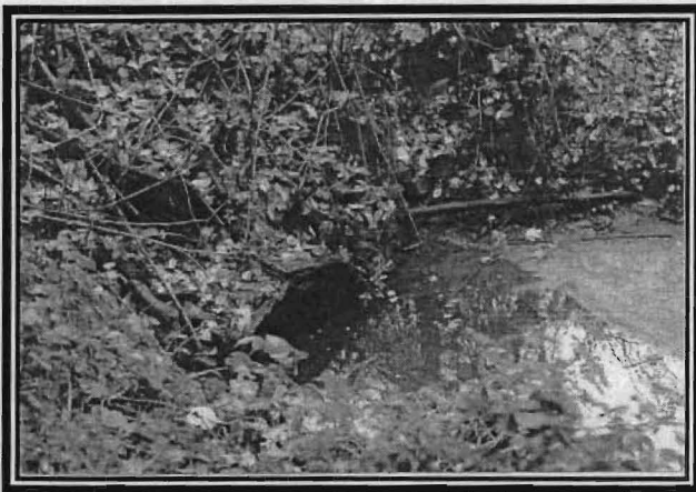
Figure 3. Spring Garden Creek culvert at Taylors Ferry and 26th Street.
