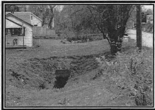
Figure 2. Streets, culverts and residential development constraining Spring Garden Creek.
